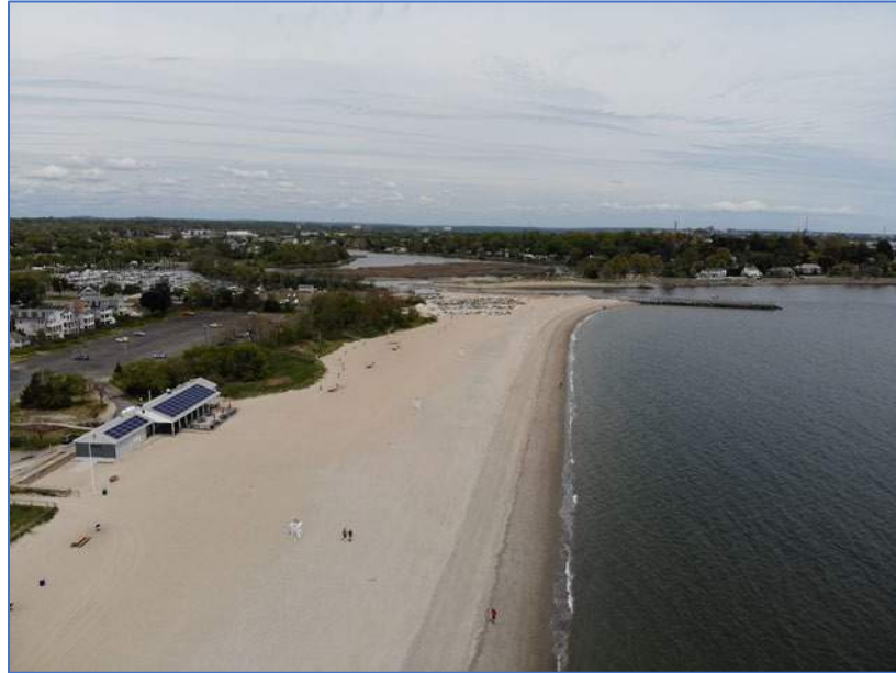
Figure 14: Beach Nourishment After Construction
