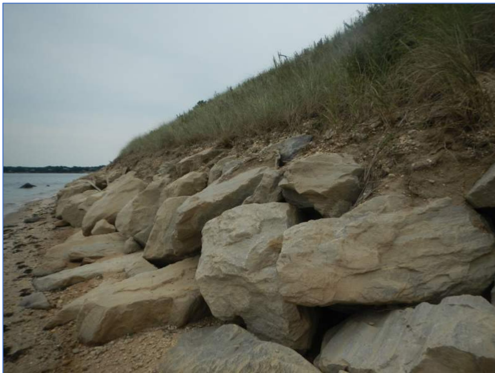
Photograph 12: Rock Revetment - Structure Type (Sheet 2 of 3)
