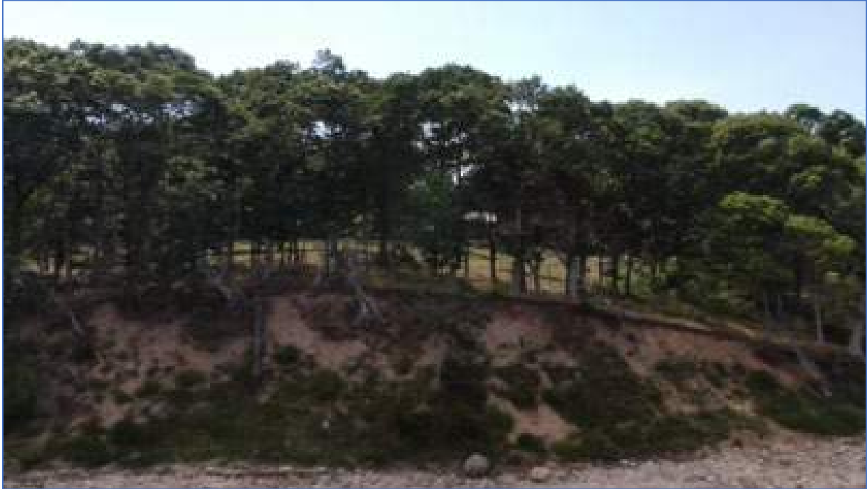
Photograph 27: Critical – Shoreline Condition (Sheet 3 of 3)
