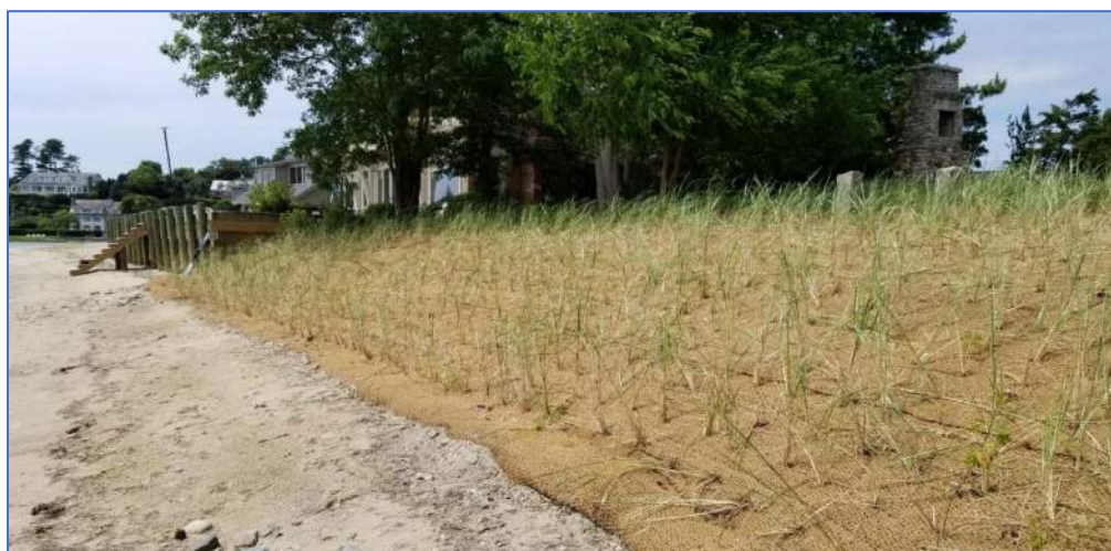
Figure 12: Coir Log Revetment with Beach Nourishment and Plantings
