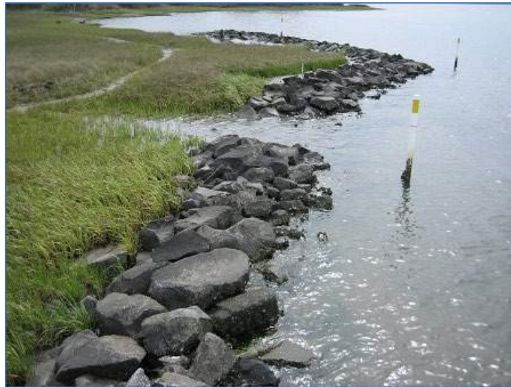
Figure 9: Rock Sill with Established Marsh
