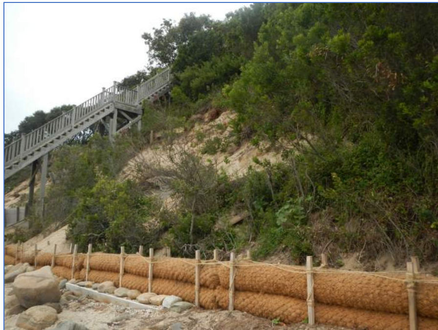
Figure 10: Coir log toe protection near On the Bluff Road
