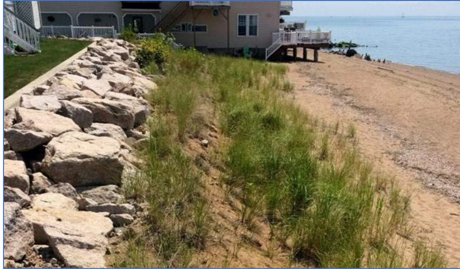
Figure 16: Hybrid Rock Revetment
