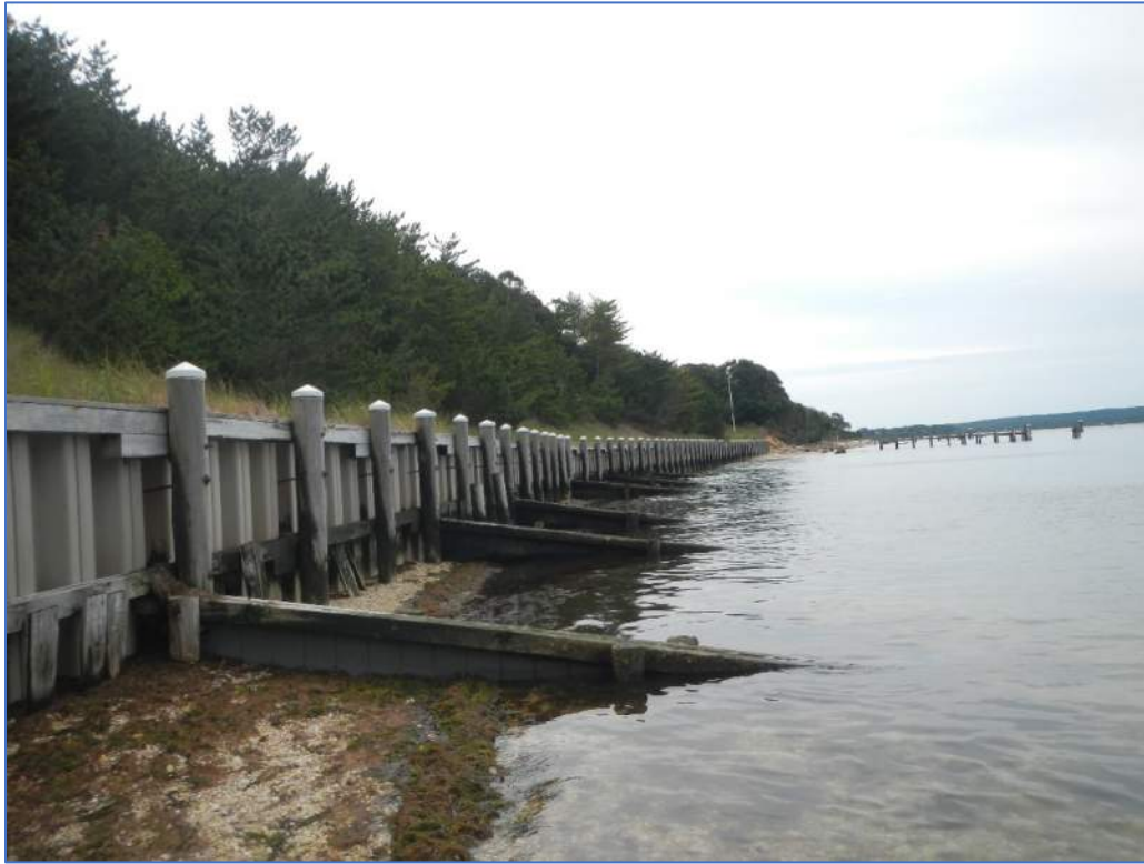
Photograph 13: Bulkhead - Structure Type (Sheet 2 of 3)
