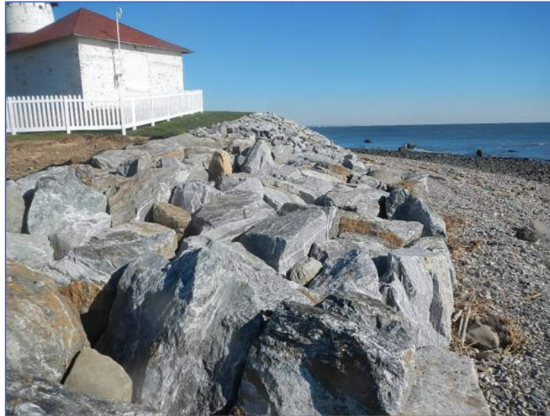
Figure 7: Rock Revetment
