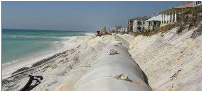
Figure 15: Geotube Reinforcement
