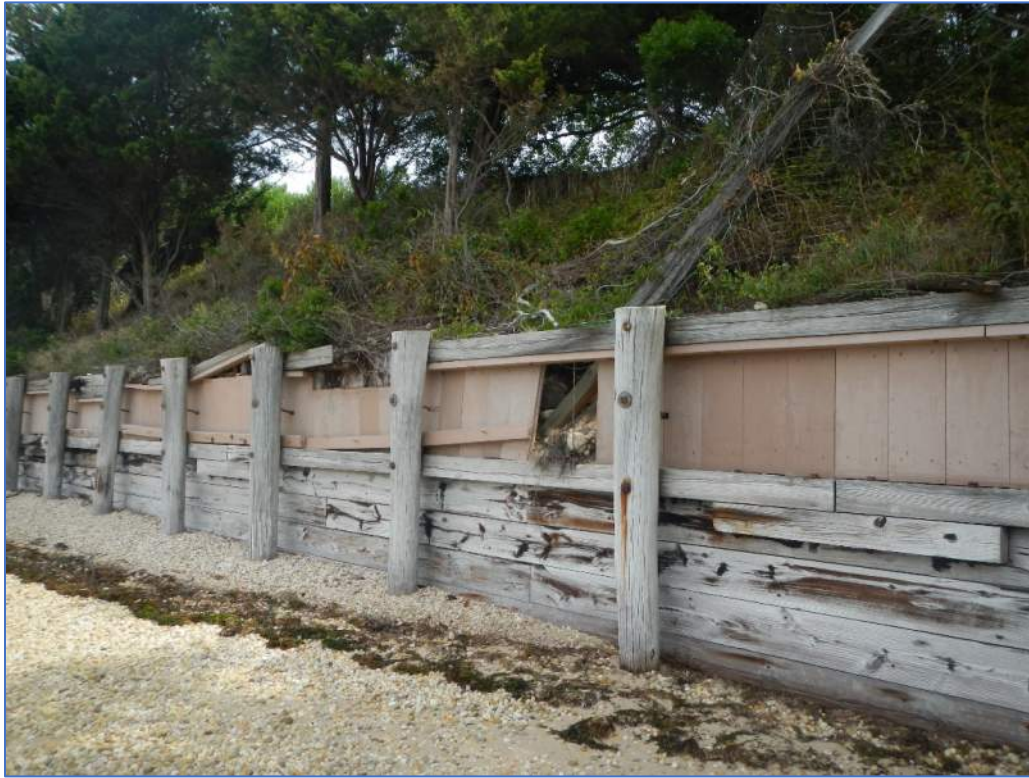
Photograph 23: Fair – Shoreline Condition (Sheet 3 of 3)
