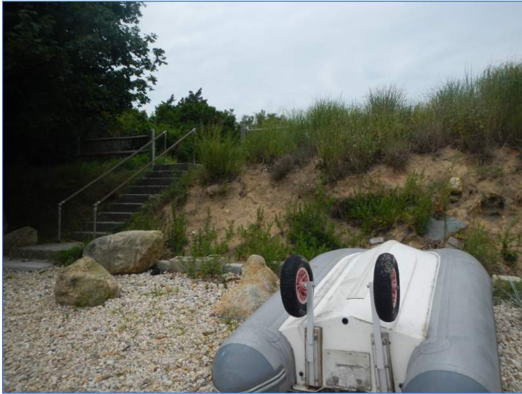
Photograph 25: Eroded – Shoreline Condition (Sheet 3 of 3)
