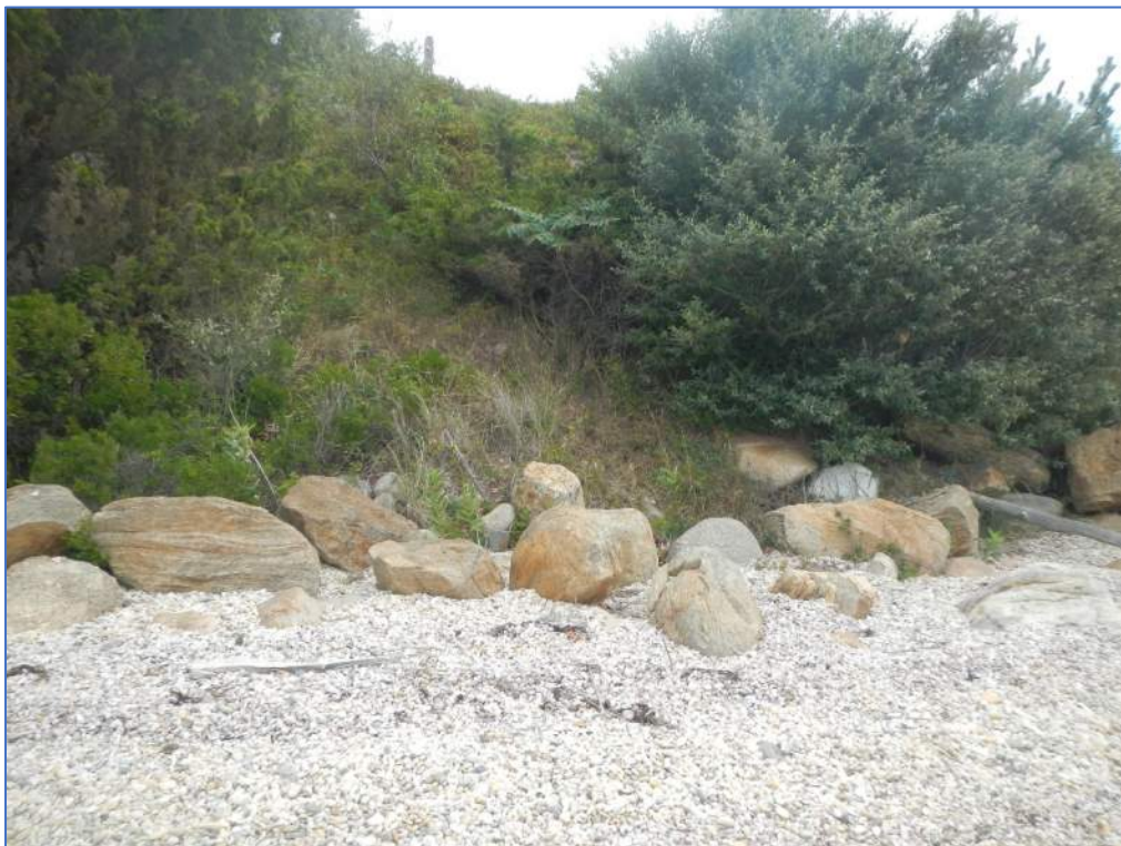
Photograph 20: Other (Random Rip Rap) - Structure Type (Sheet 2 of 3)
