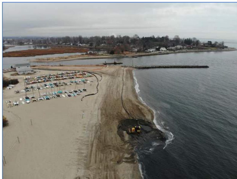
Figure 13: Beach Nourishment During Construction
