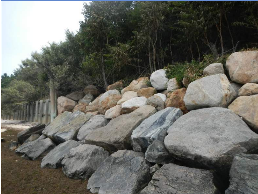
Photograph 11: Rock Revetment - Structure Type (Sheet 2 of 3)
