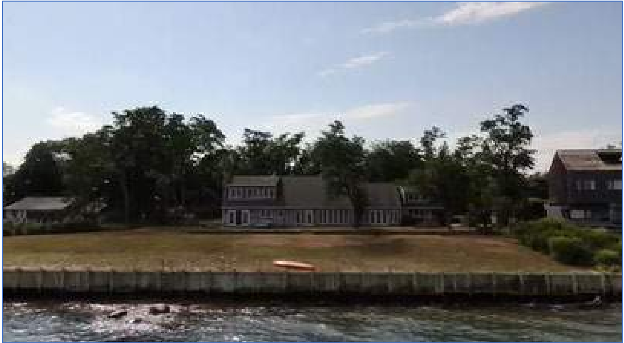
Photograph 9: Other (Water Against Bulkhead) - Shoreline Type (Sheet 1 of 3)
