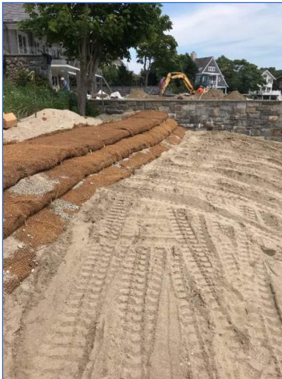
Figure 11: Coir Log Revetment Under Construction
