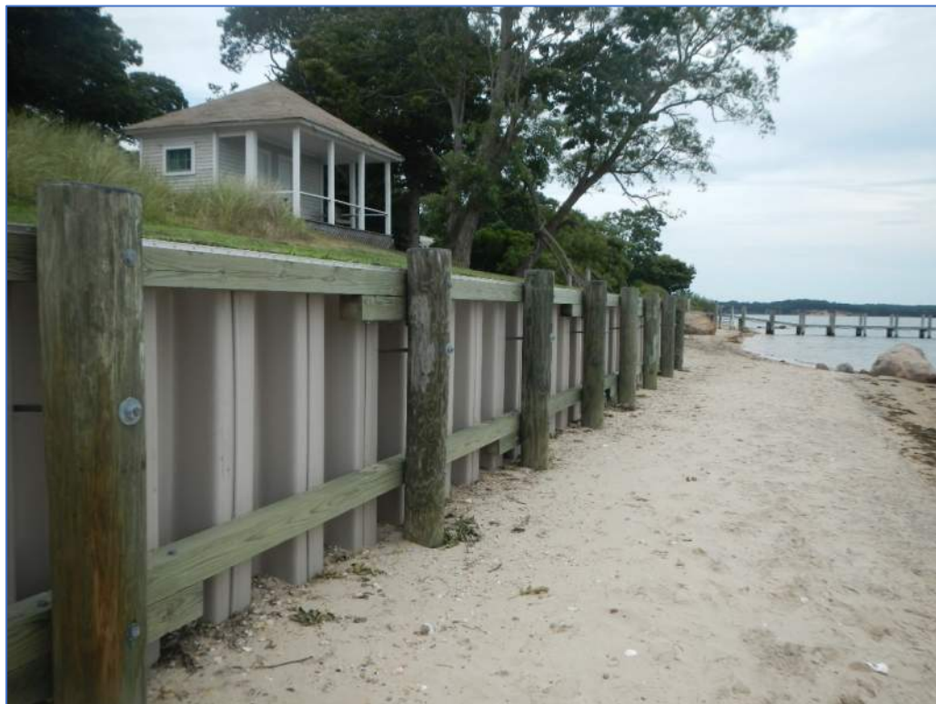
Photograph 14: Bulkhead - Structure Type (Sheet 2 of 3)
