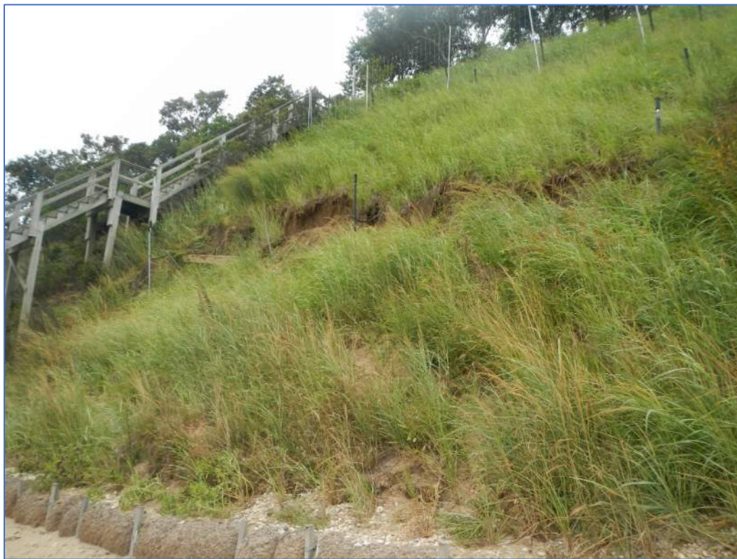
Photograph 24: Fair – Shoreline Condition (Sheet 3 of 3)
