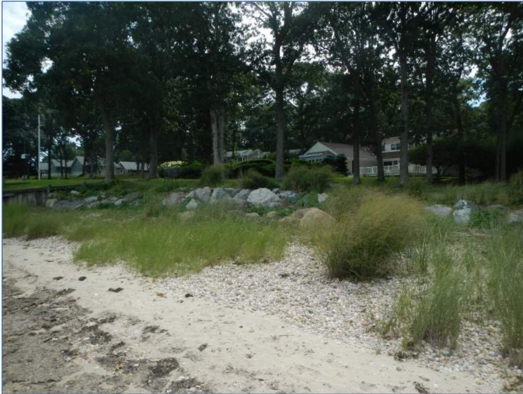
Photograph 19: Other (Random Rip Rap) - Structure Type (Sheet 2 of 3)
